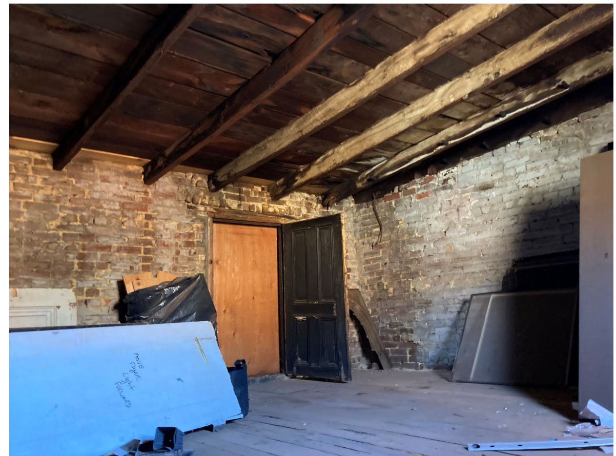
EXISTING ATTIC OF GARAGE
