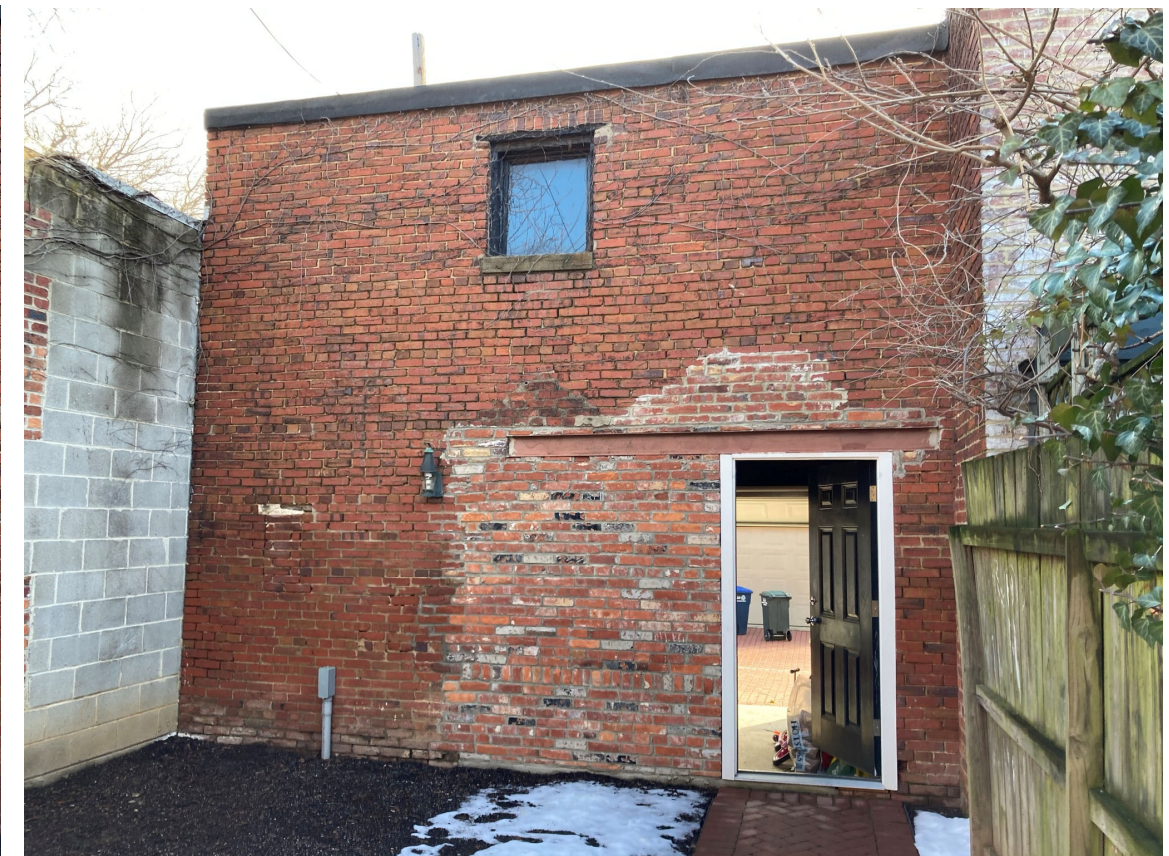
YARD FAÇADE OF EXISTING GARAGE
