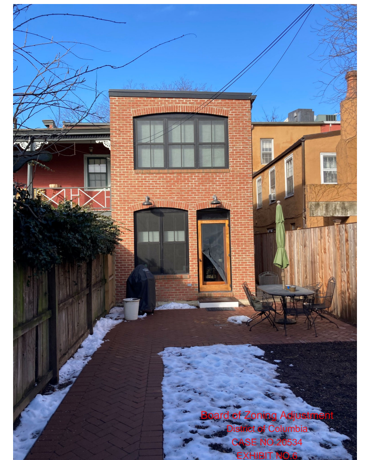
EXISTING REAR FACADE
